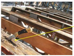
Decayed timber is soft and spongy and can easily be penetrated with a knife or screwdriver
