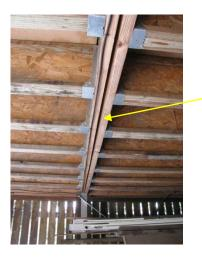
Expansion of the hardwood T&G floor above has caused the separation of double bearers.
